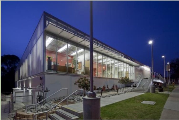
“P” Building Renovation
