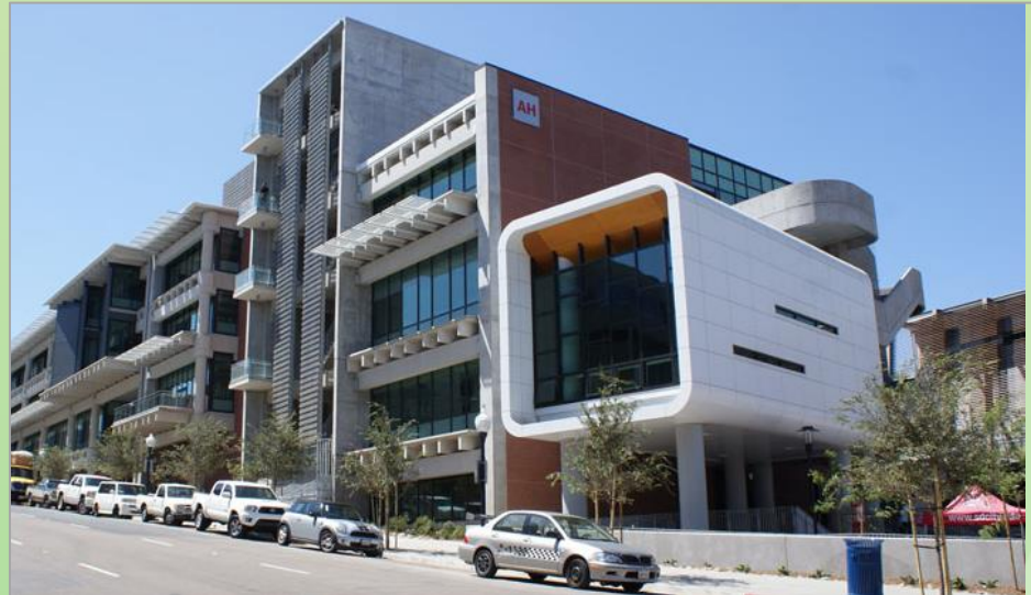
Arts and Humanities Building
