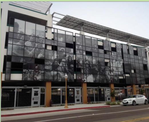
Cesar Chavez Parking Structure
