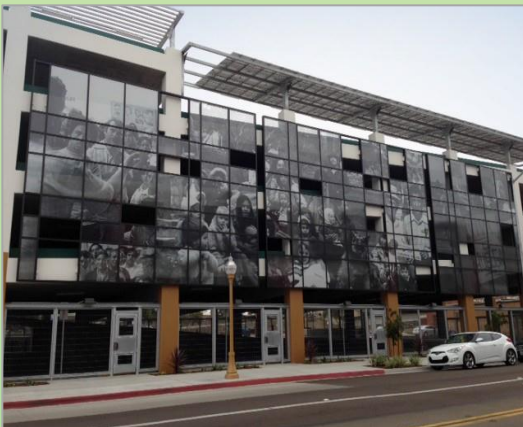
Cesar Chavez Parking Structure
