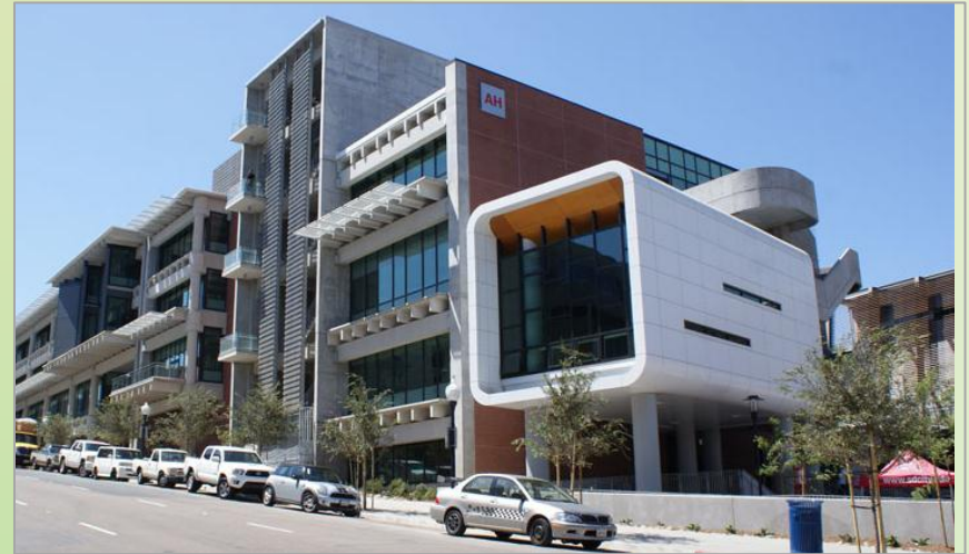
Arts and Humanities Building
