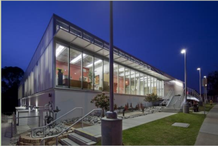
“P” Building Renovation
