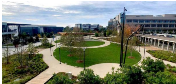
San Diego Mesa College's final bond project — the campus Quadrangle — is the final major project in the Propositions S and N bond construction campaign.
